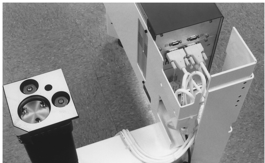
Figure 2.5 — Installing the Controller and Cabling
