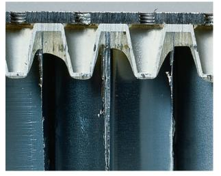
Figure 15: Cross-section view of Newport's cup design.
